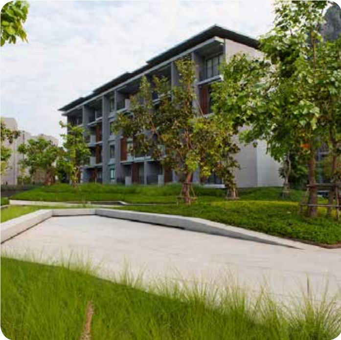
Graded planting areas
